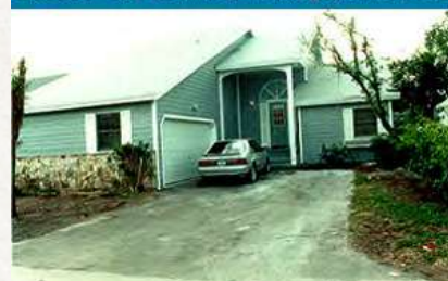
Level 2 - Major damage; habitable
